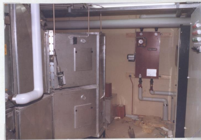
31.3.84 Varmefordelingsrom under taket.
